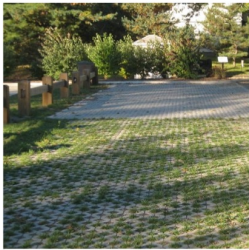
Grass and Grid Pavers (Hole in the Wall Parking Lot, East Lyme, CT)
