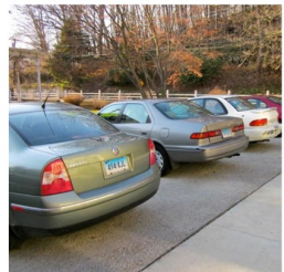
Pervious Concrete (Residential Subdivision, East Haddam, CT)
