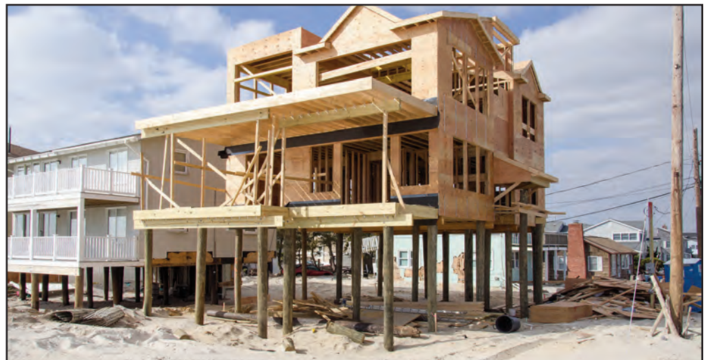
Signs of recovery from Hurricane Sandy in the form of new construction, elevated to the new standards, are seen in Beach Haven, NJ. Photo by Liz Roll/FEMA
