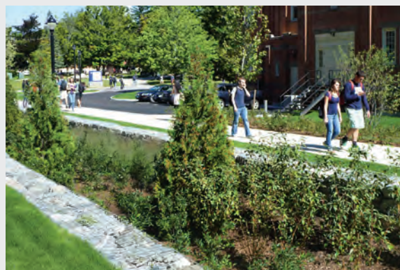
Students walk by a large bioretention basin behind Oak Hall, Storrs, CT.
