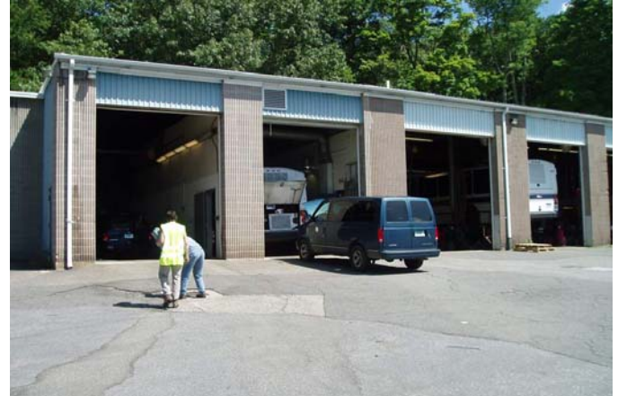
Figure 2. Motorpool parking lot (top) and existing external
