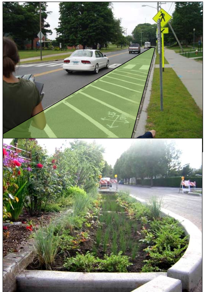
Figure 2. Remove pavement along existing road shoulder to edge of existing curb (top). Example street planters with curb cuts from Portland, OR (bottom).
