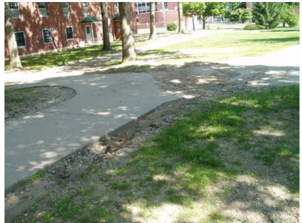
Figure 1. Runoff from quad walkways resulting in erosion (top); Sediment accumulation on walkways and in quad area (bottom).
