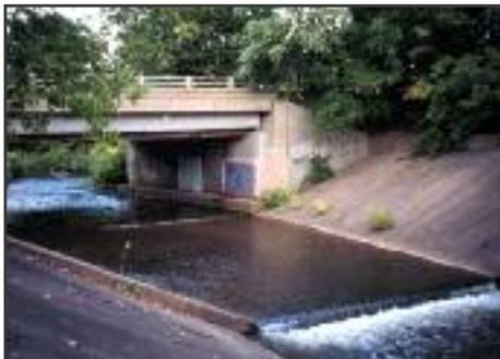
As development increases in a given watershed, changes occur to the water quality and quantity of the receiving stream. (Top) Streams in less developed watersheds typically exhibit a meandering form with banks stabilized by vegetation. (Bottom) Streams in highly urbanized areas often need to be channelized to control flooding and erosion problems resulting from large pulses of stormwater.
