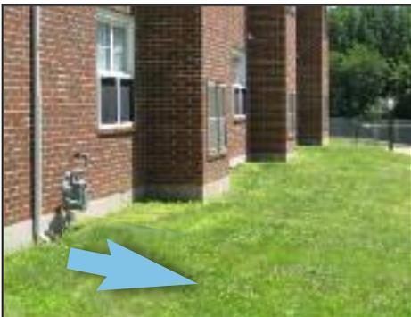
An important distinction when dealing with impervious cover is whether it is *connected* or *disconnected*. (Top image) A parking lot which is directly connected to the drainage system, which flows into a nearby stream. (Bottom image) Runoff from the impervious rooftop is channeled via the leader into an extensive lawn area where the water can infiltrate, effectively disconnecting this portion of the roof from the drainage system.
